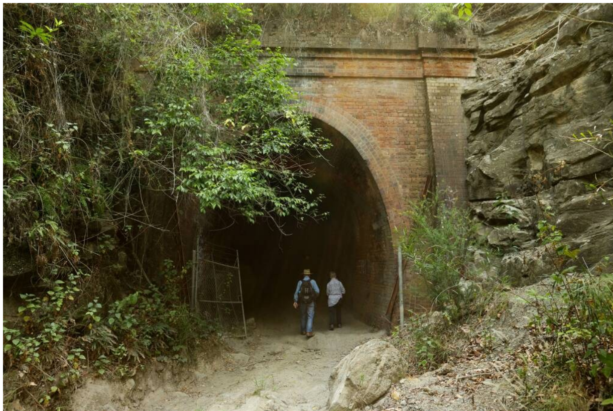
A tunnel on the proposed Richmond Vale Rail Trail. Picture: Jonathan Carroll
