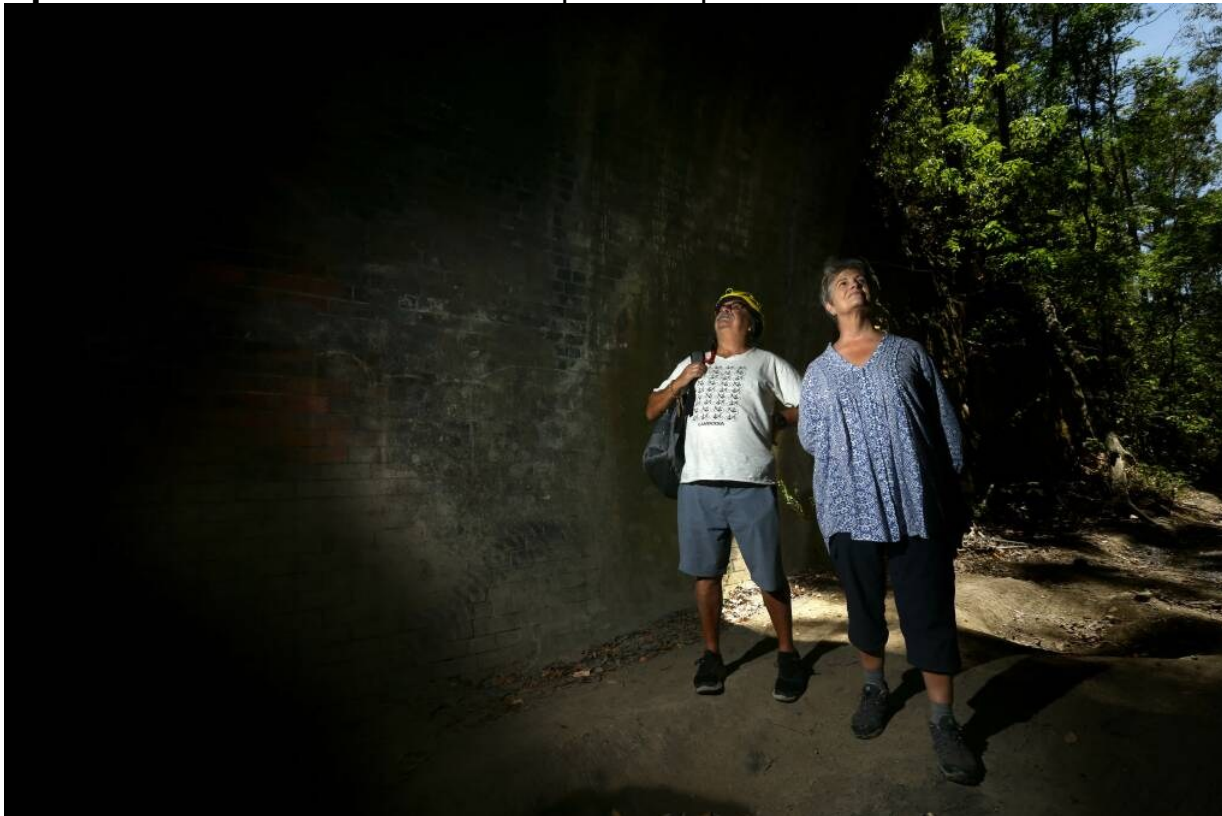
TUNNEL VISION: Billy Metcalfe and Leigh Gibbens inspect the historic No.1 Tunnel on the former Richmond Vale Railway. Picture: Jonathan Carroll
