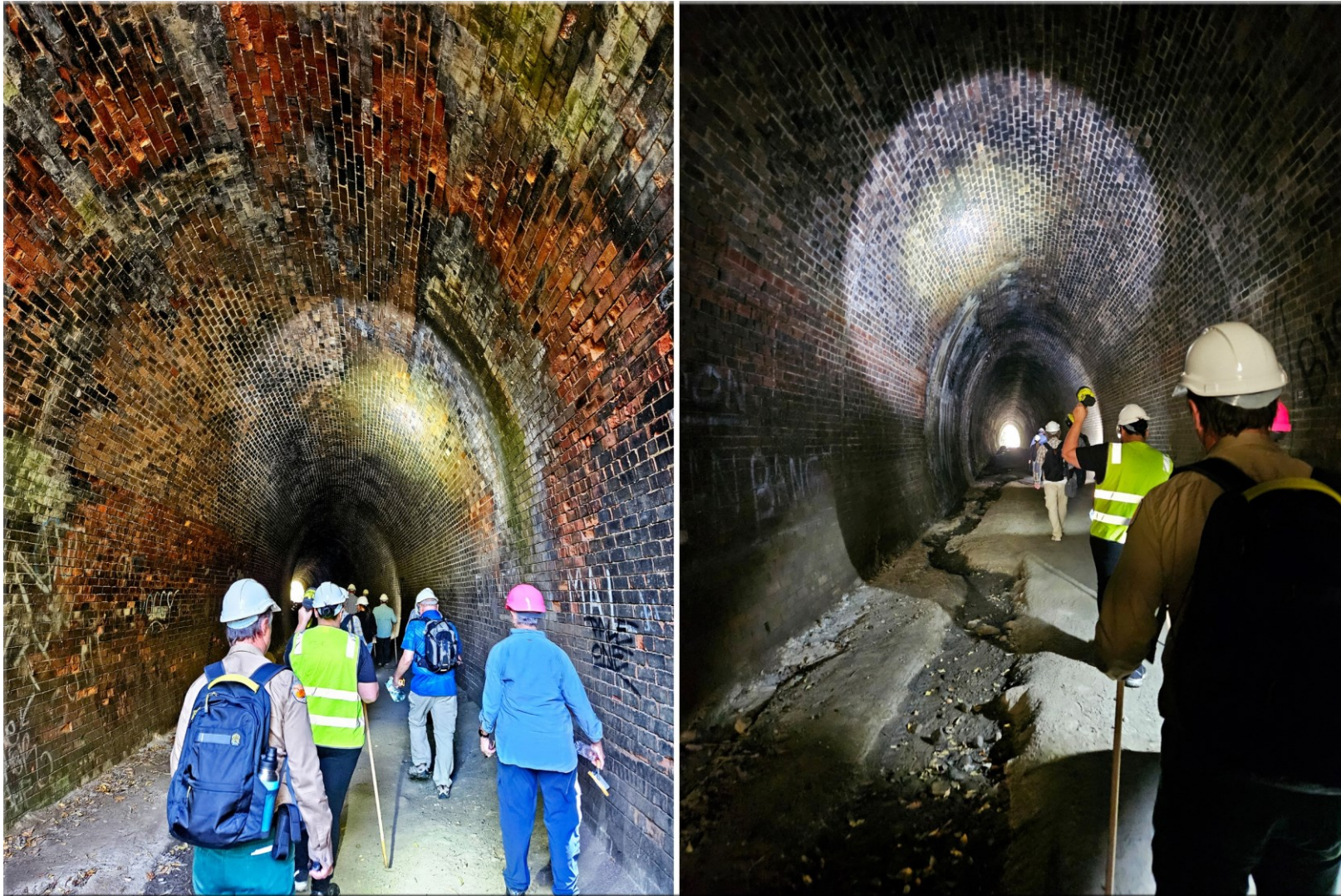
Image 7. Walking in an Easterly Direction through Tunnel #1 (Sept. 29 th 2023) – a 160m Brick-lined Tunnel Opened in 1905 as part of the Richmond Vale Railway.
