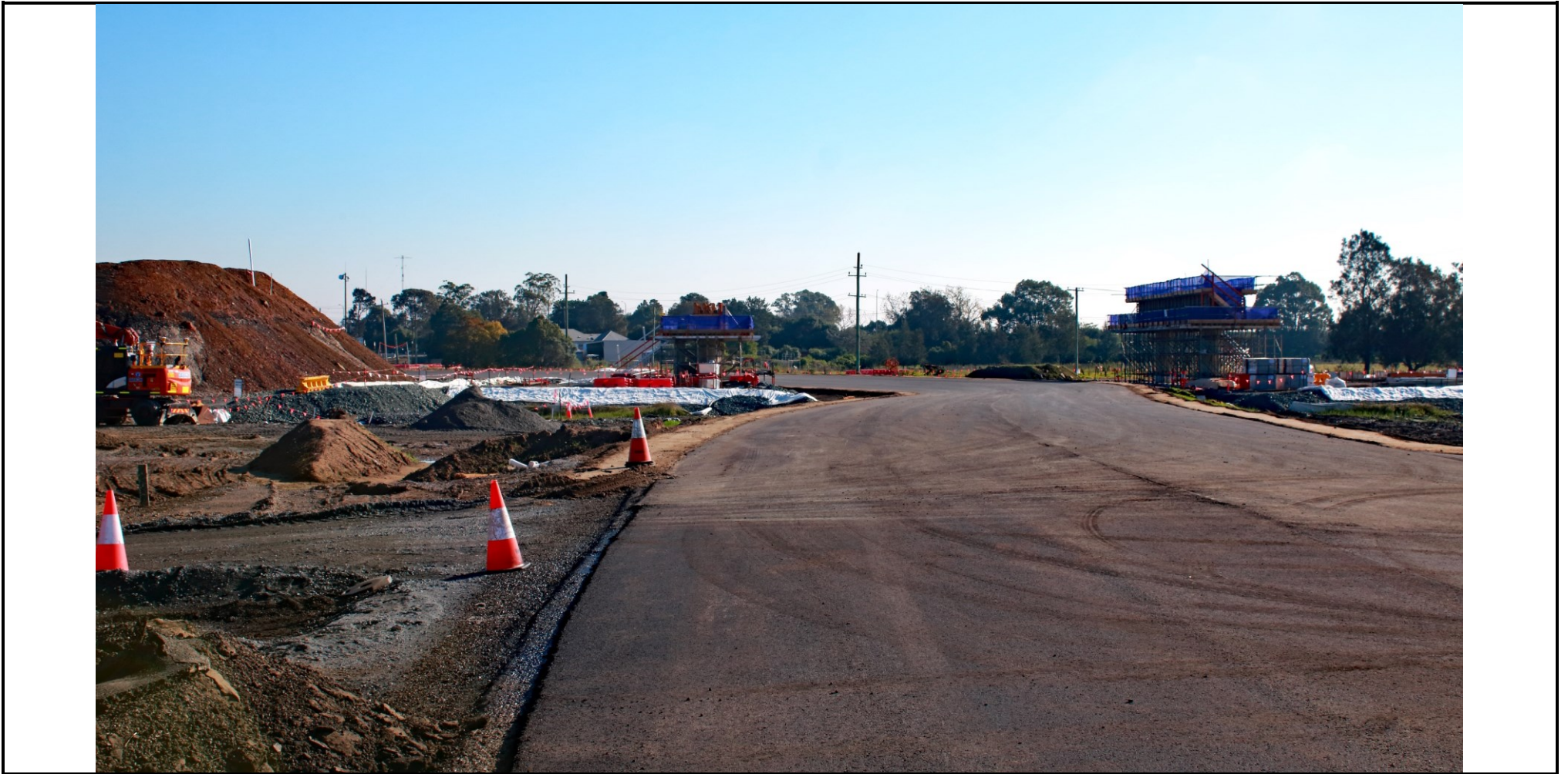
Picture 6: Partially Sealed Re-located Aurizon Access Road (Tarro) – May 26th 2024.
