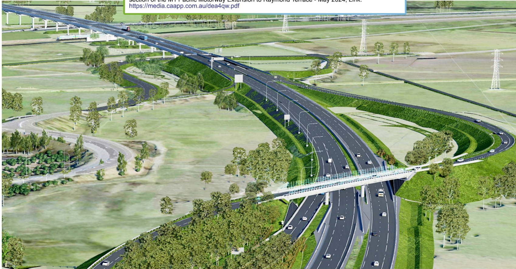
Figure 105: Aerial view of BR06 - looking east
