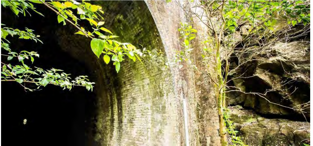
Figure 1-3 Tunnel 2 near Blue Gum Creek
