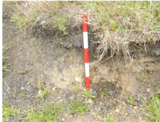
Figure 170: Sandy soil located in erosional ground exposure near base of embankment. South aspect.
