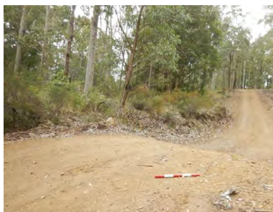
Figure 166: View of access track rollover, east aspect
