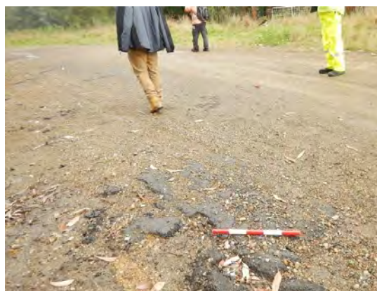
Figure 134: Remnant bitumen from former Seahampton Road sealed road surface, west aspect
