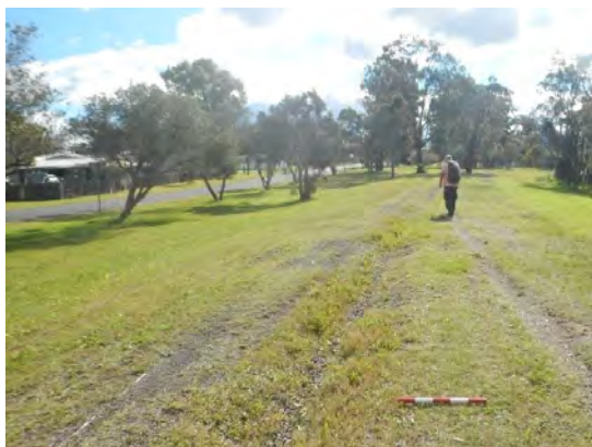
Figure 102: Raised embankment and ashy soil of former rail line, Pelaw Main. North west aspect.
