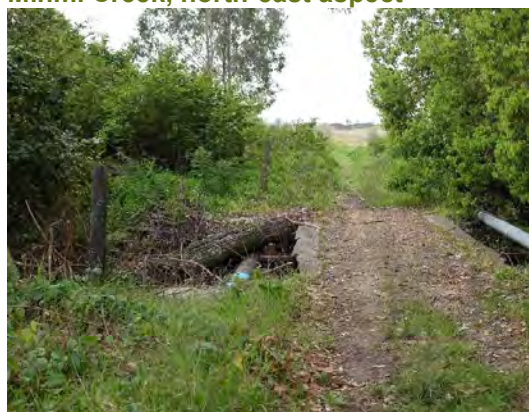
Figure 53: Concrete culvert and bridge over Minmi Creek, north-east aspect
