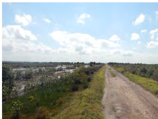
Figure 23: Pipeline Road and supporting embankment, north aspect
