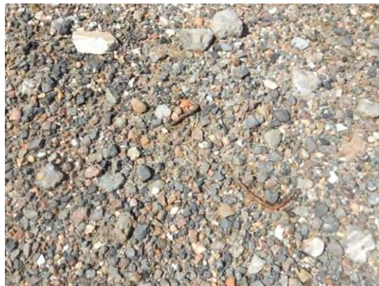
Figure 25: Imported fill to construct the Pipeline Road embankment
