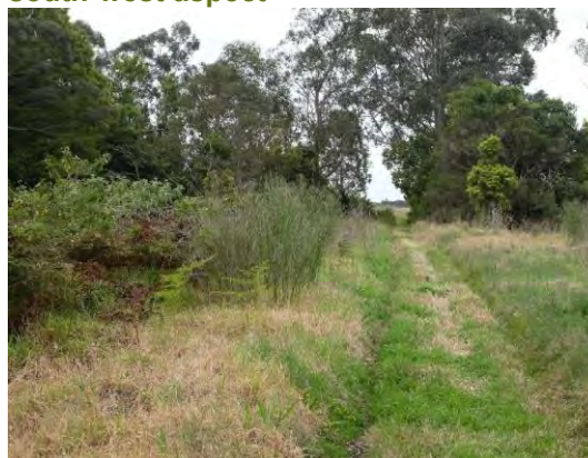
Figure 55: Grass cover on Minmi to Hexham railway line in southern portion of survey unit, south-west aspect
