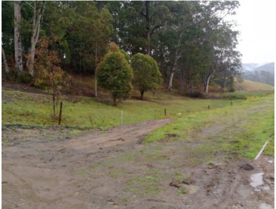
Figure 60: Washed in sediment over the rail route, west aspect
